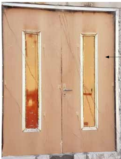
Single acting double door with steel frame
